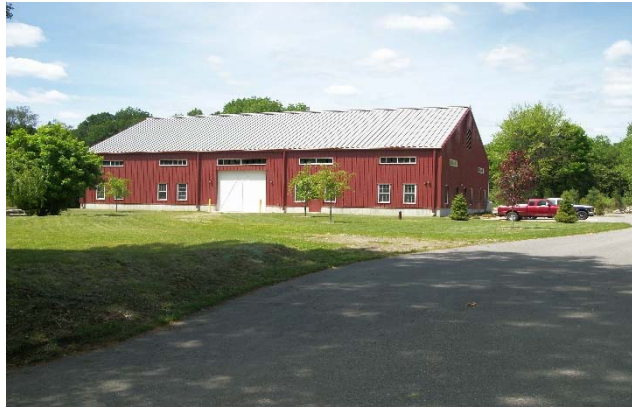
The new Hampton Public Works Garage
